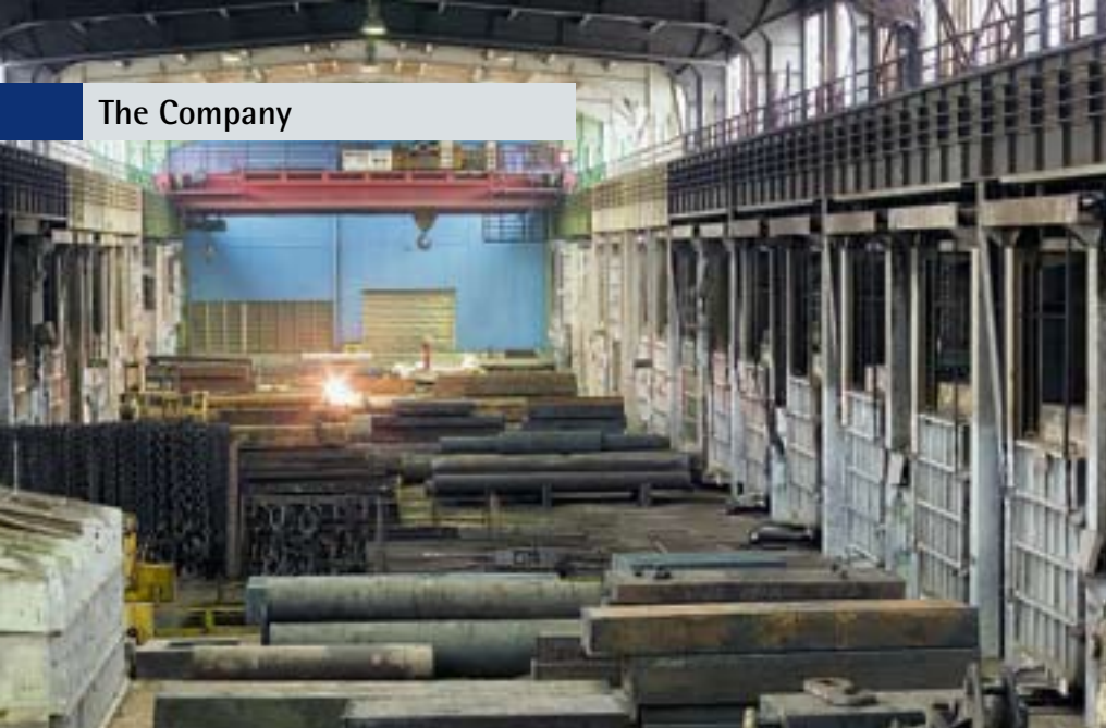
Overall view of the annealing shop
