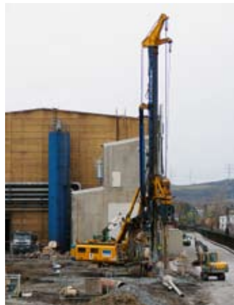
Rotary boring machine in action
