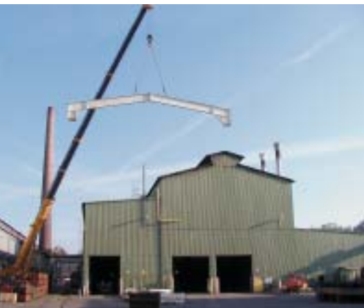
Converting the forging shop roof
