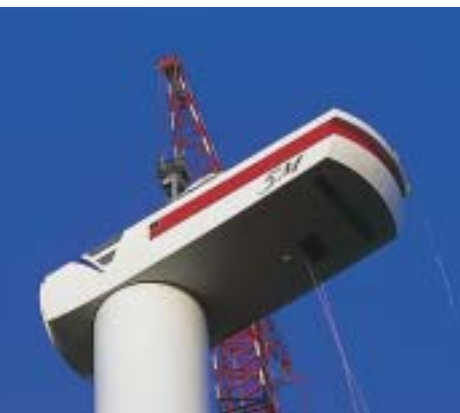
The machine housing comprising gear steel from Wetzlar is assembled on the ground – The complete power house is fitted in one piece – The complete 5M wind power generator (from left to right)
